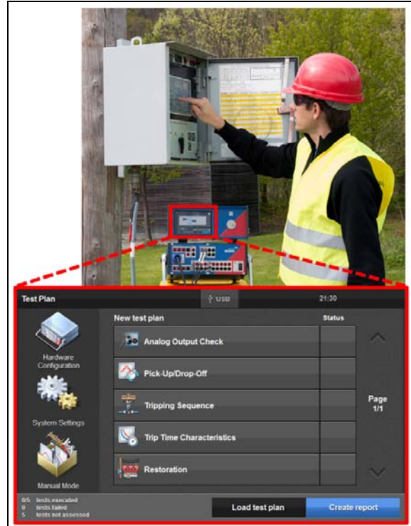
Fig. 7 Engineers conduct on-site test on recloser controls with prepared test plans on CMControl
